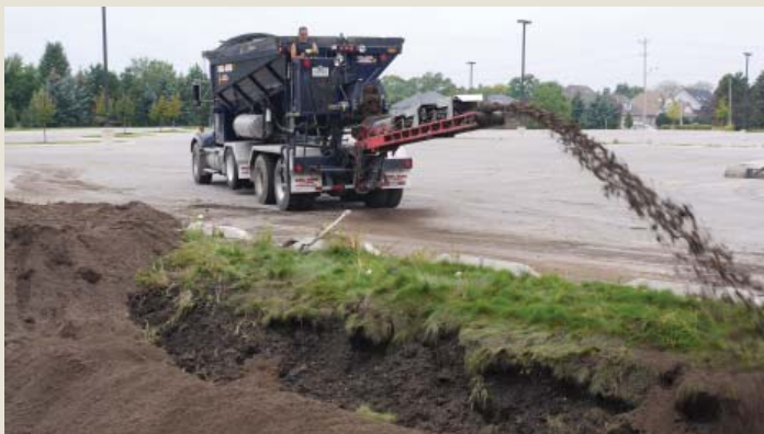
Slinger truck evenly placing bioretention soil in a large cell
