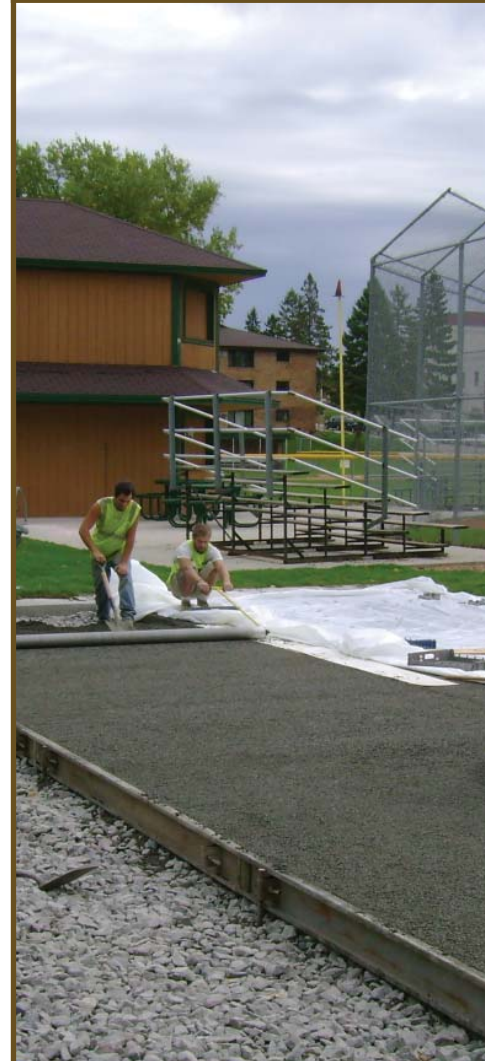
Top: roller compaction Lower: plastic placement
