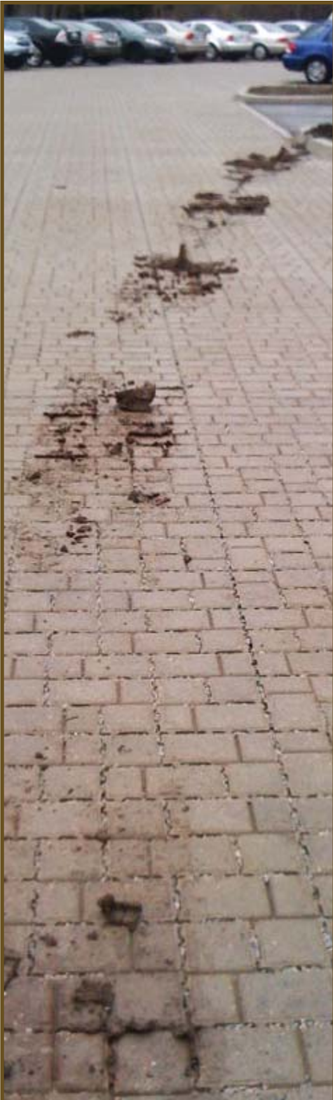
Tracked sediment on permeable pavement.
