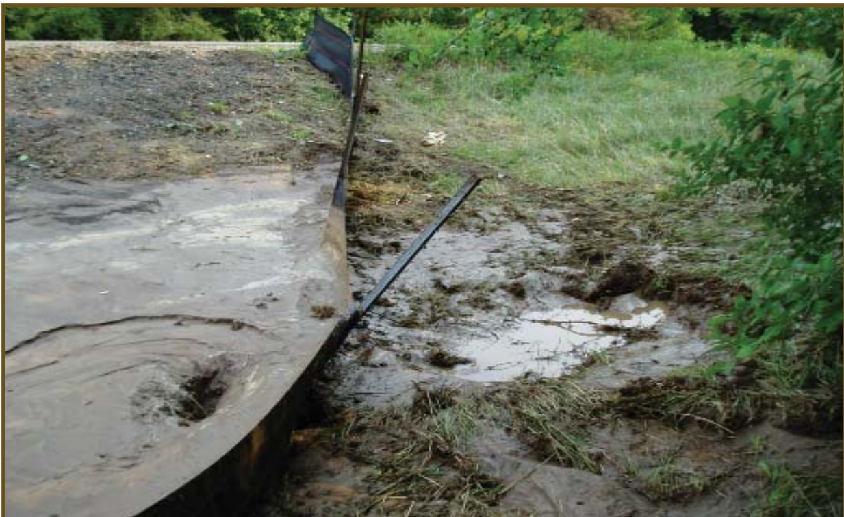
Failure at a single point of a perimeter control - see ESC Guide for maintenance scheduling
