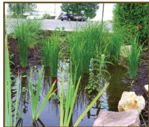
BMP holding water longer than design drawdown time
