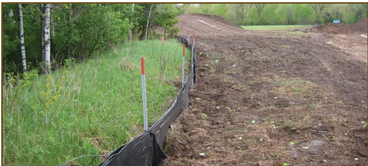
Preparation of pedestrian, nature trail with proper erosion control established during construction.
