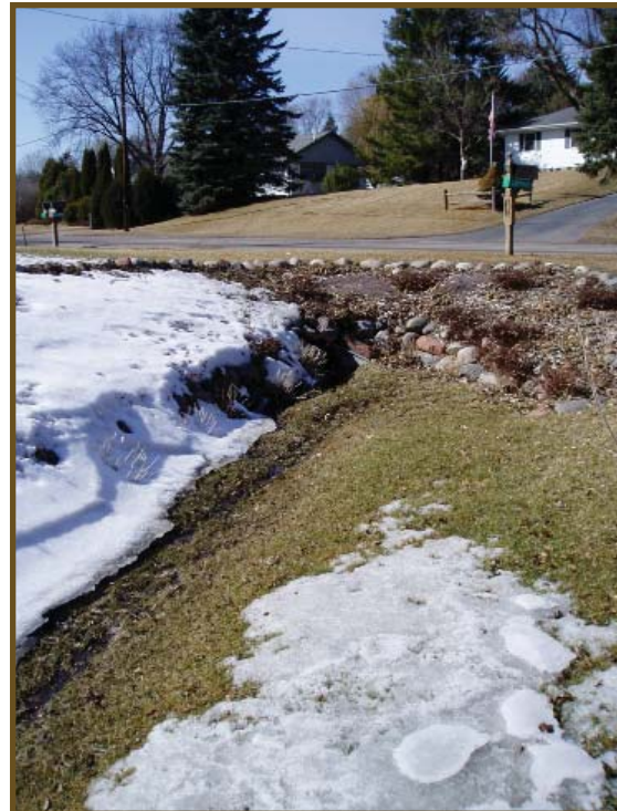
Spring melt can contribute to the sedimentation and reduced performance of BMPs.
