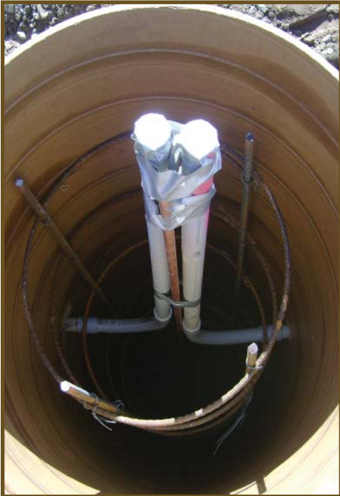
Lighting base installation.
