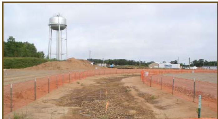
Caution fencing prevents traffic and building materials storage within the BMP.
