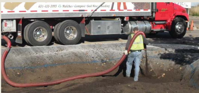
Pneumatically applied bioretention soil medium (Source: Windscaapes)
