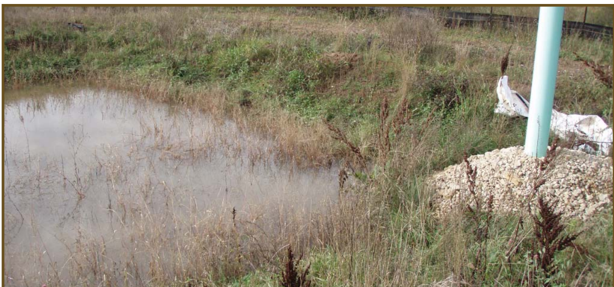
Temporary Sediment Basin
