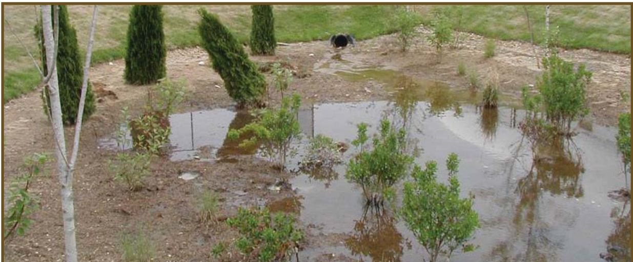
Bioretention clogged with construction sediment which could have been prevented with an effective ESC report and implementation. Source: LID Center
