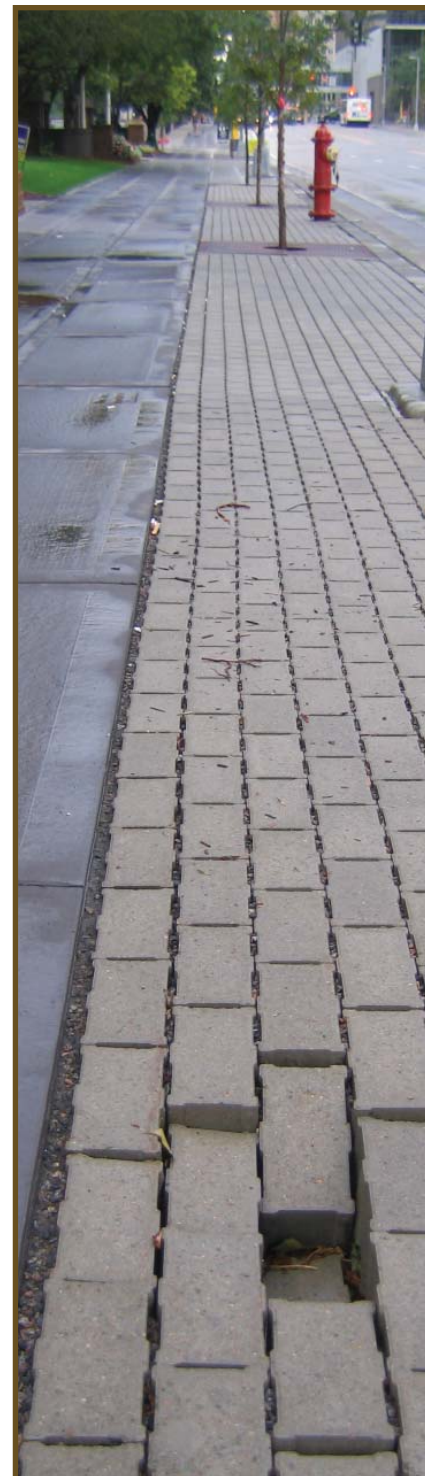
Uneven settling caused failure of these pervious pavers that were used in a heavy traffic, urban setting.
