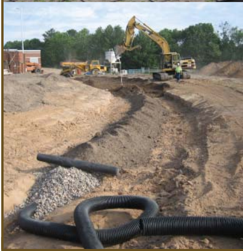
BMPs in construction: Top - underground storage units Middle - green roof installation Lower - infiltration trench
