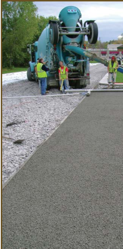
Installation of pervious concrete; community recreation application.
