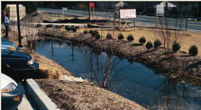
Unanticipated soil settlement resulted in increased ponding depth (Source: LID Center)
