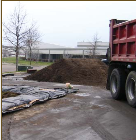
Top: concrete washout next to future BMP - poor location
