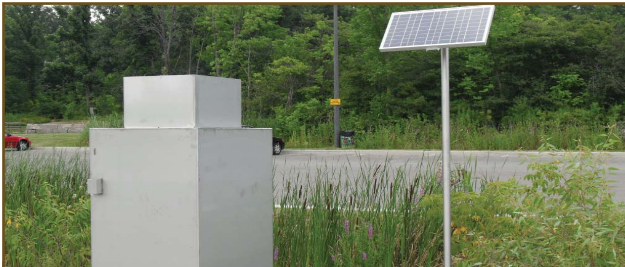
Bioretention monitoring station.
