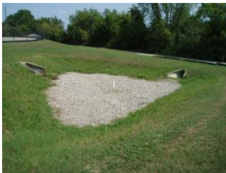
Figure B-8. Photo of Infiltration in Good Condition
