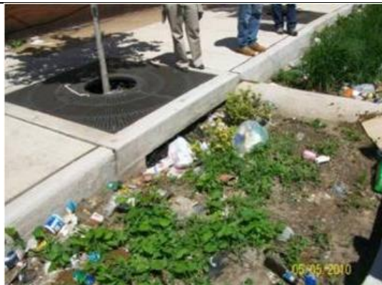
Bioretention full of trash and needs to be cleaned out.
