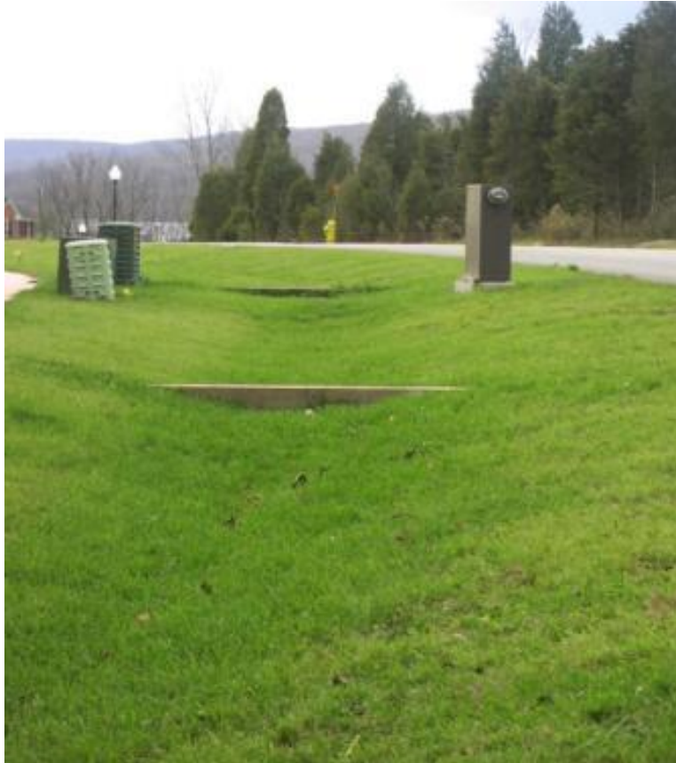
Figure B-2. Photo of a Grass Channel in Good Condition
