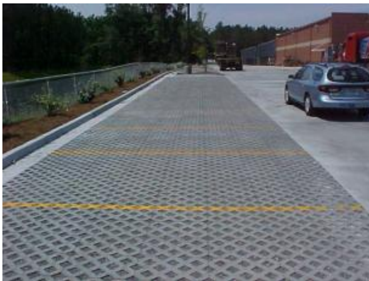
Figure B-6. Photo of Permeable Pavement in Good Condition
