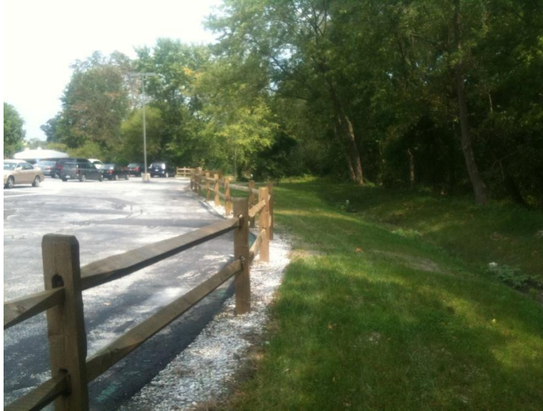
Figure B-4. Picture of a Filter Strip in Good Condition
