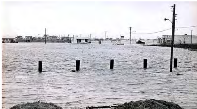
Figure 2: Flooding in Lewes during the 1962 Ash Wednesday Storm.
