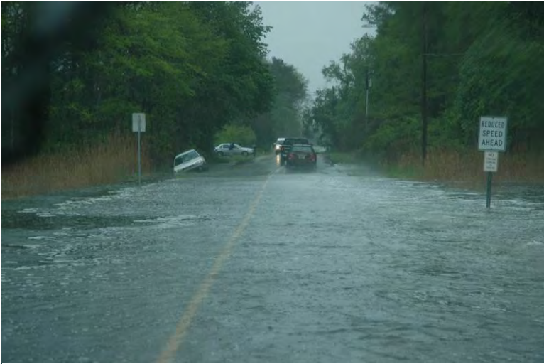
Figure 3.1: Flooded roadway (New Road) during 2008 northeaster.
