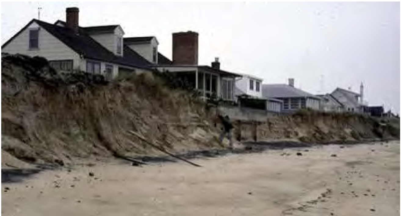
Figure 3.10: Erosion along the Delaware Bay shoreline, Lewes Beach.
