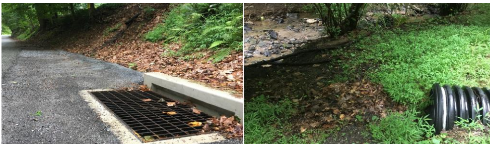
Left: Street inlet; Right: Outfall pipe discharging directly to a stream.
