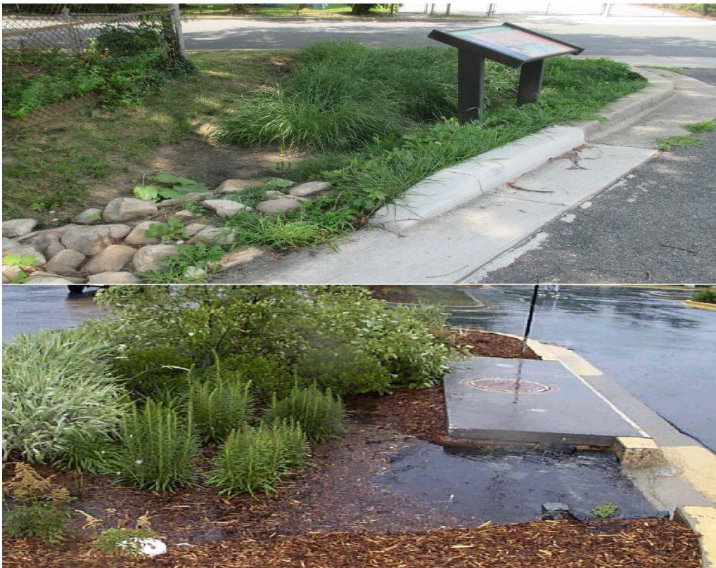
Top: Rain garden at City Hall, Edmonston, MD. Bottom: Bioretention retrofit, added to existing parking lot islands with conventional inlets. Source: www.ence.umd.edu/~apdavis/Bioinstallations.htm
