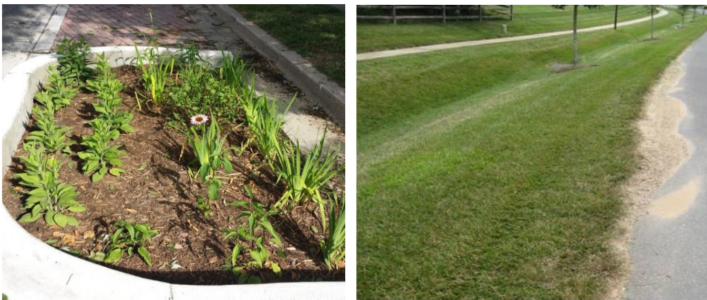
Left: Rain garden, City of Cambridge, MD; Right: grassed swale; source: chesapeakestormwater.net/wp-content/uploads/2014/06/UFS2.jpg
