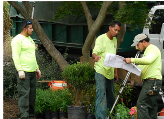
A well-prepared crew consults a full-size printed drawing during plant installation.
