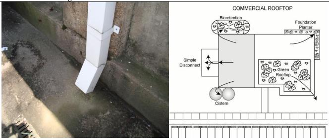
The **left panel** shows a typical roof downspout that discharges to a paved surface and then into a storm drain. These directly connected downspouts do not allow for any treatment of stormwater before it is discharged to the stream. The **right panel** shows a wide range of options for disconnecting and treating roof runoff, from simple disconnection over a pervious area to rain tanks that reuse stormwater and increase plant water efficiency.
