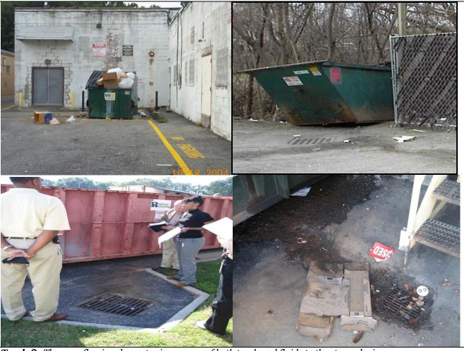
**Top left:** The over-flowing dumpster is a source of both trash and fluids to the storm drain **Bottom left:** Note the stain lines between the open dumpster containing used metal products and the storm drain inlet. **Top right:** The direct leakage of dumpster juice into the storm drain could have been prevented by simply moving it to another site location. **Bottom right:** Compactors that compress materials with fluids can be a chronic problem when connected to the storm drain system
