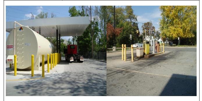
This fueling area on the **left** has been designed with a cover to keep rainwater away from any spilled diesel, and also has a spill response kit. Contrast this with the uncovered fueling area on the **right**, with obvious petroleum stains that reach the storm drain system
