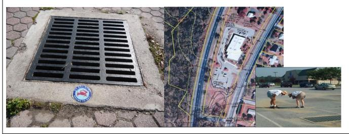
The survey is best done when it is raining, and should also pinpoint the location of storm drain outfalls which may be located off the site (**right**). Once you are done with the survey, make sure to mark all storm drain inlets "Keep pollutants out- drains to X stream or river" (**left**)so that employees understand that they are stormwater inlets and are not connected to the wastewater treatment plant.
