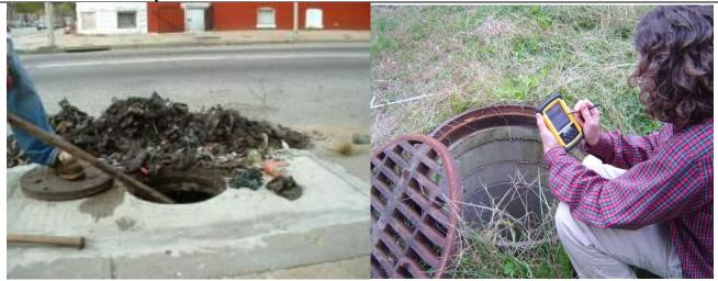
By removing trapped sediments in your storm drain infrastructure you keep these pollutants from eventually reaching the stream (left). Storm drain inlets and stormwater practices should be visually inspected at least once a year to identify any maintenance tasks that are needed to assure the continued performance and longevity of the stormwater infrastructure (right)
