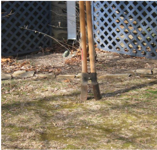
Post Hole Digger for Soil Test
