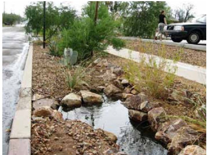
Curb inlet allows stormwater runoff to enter a street-side basin
