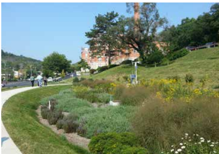
Completed bioinfiltration basin project at the St. Francis Court Apartments, adjacent to the Lick Run Project corridor
