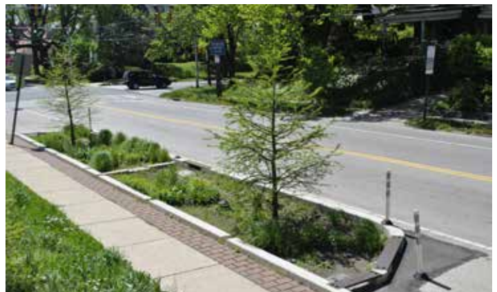
Stormwater bump-out outside the Queen Lane Drinking Water Treatment Plant in Philadelphia
