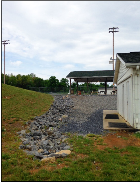
Stormwater management in Oatesdale Park
