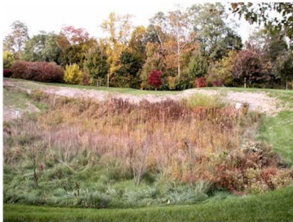
FIGURE 5-43 Dry extended detention pond. SOURCE: PaDEP (2006).
