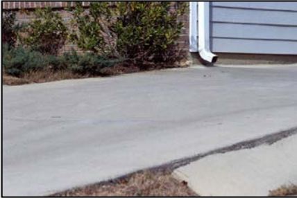
A directly connected roof drain
