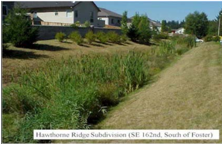
FIGURE 5-16 Vegetated swale. SOURCE: PaDEP (2006).
