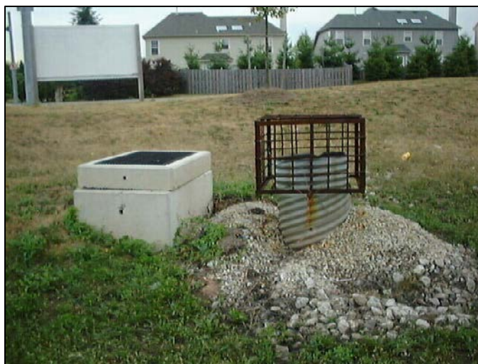
FIGURE 5-8 Sediment filter left in place after construction. SOURCE: Robert Traver, Villanova University.
