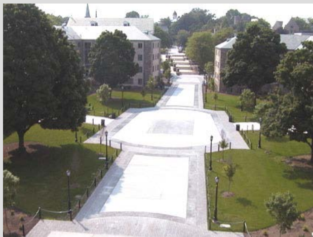
FIGURE 5-33 Villanova University pervious concrete retrofit site. SOURCE: Reprinted, with permission, from VUSP. Copyright by VUSP.
