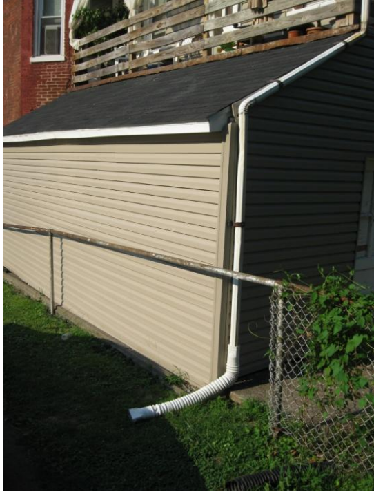
Residential downspout disconnection in Lancaster, PA
