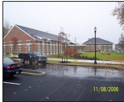
Porous asphalt parking lot in Wilm., DE
