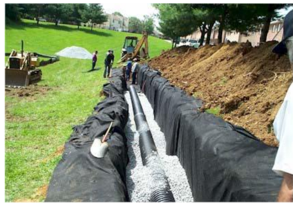
Infiltration trench Chester County, PA
