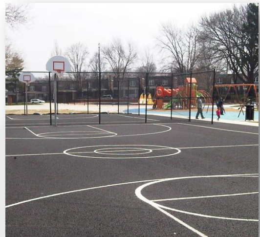
A porous basketball court at 6 th Ward Park plan progressed from idea, to concept, to construction during the development of the GI Plan.
