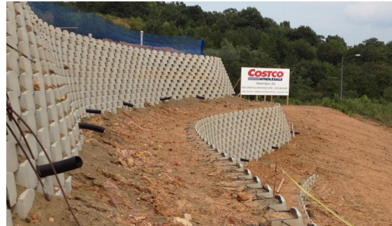
The retaining wall being installed in steep, non-porous clay earth site.
