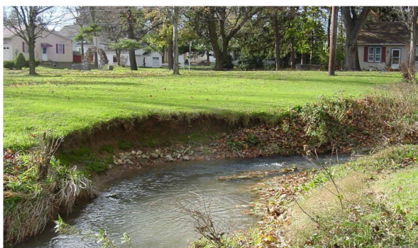
Eroding banks of Santo Domingo Creek before restoration
