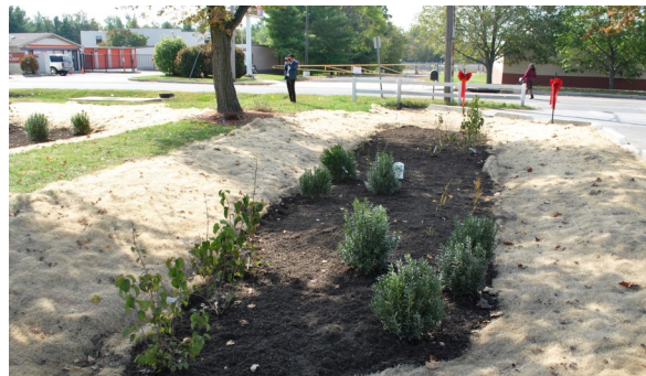
Native plant rain garden that captures and cleans thousands of gallons of polluted runoff from the parking lot
