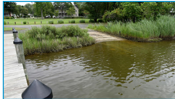
Biocells that strain runoff before it reaches the Bay
