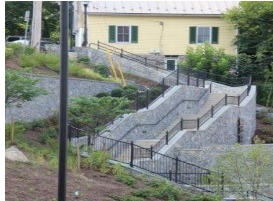
A stormwater flume connects flow from Main Street, under the stone staircase to a series of BMP's within it.
