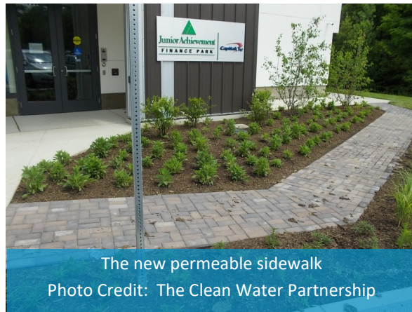
One of three new rain gardens on campus
