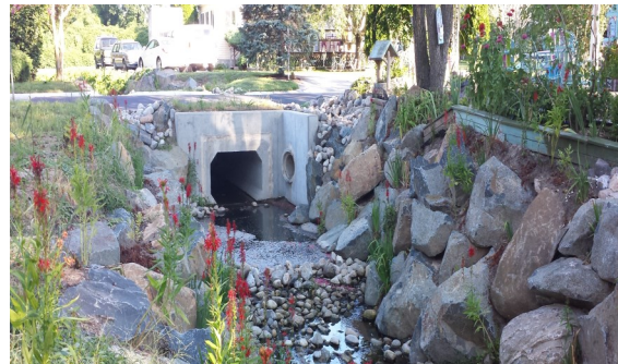
The new culvert and stream channel alleviated flooding.
