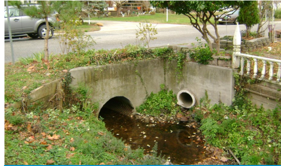
A failing culvert caused erosion and flooding in downtown Berlin.
