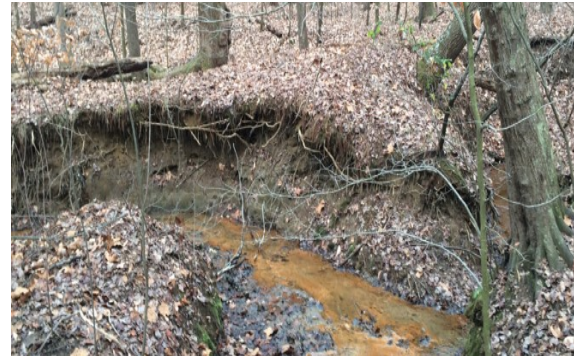
Before: The stream was becoming unstable. Headcuts like the one shown above were getting worse after each storm.
