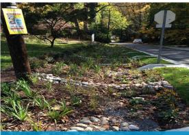
The Sligo Creek Bioretention area that replaced the old central piping solution
