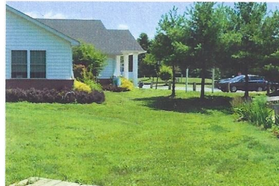
Water runoff from the roof and parking lot was flooding the school after every rain.
