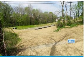
A surface sand filter with experimental flocculants corrects the drainage issues and serves as a trial run for best practices.
