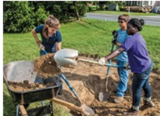
The raingarden under construction
