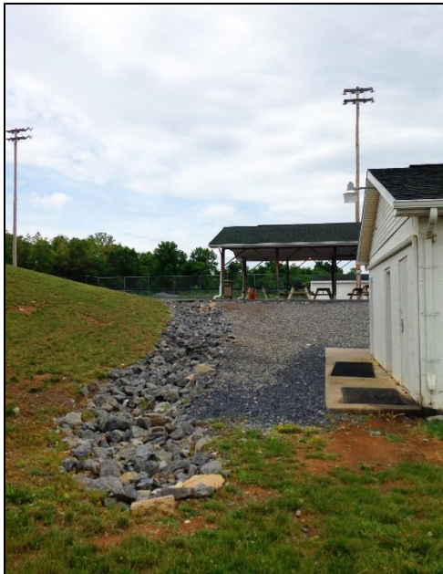
Stormwater management in Oatesdale Park
