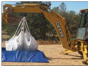
Figure 12. Extracting the concrete solids or gelled washwater
