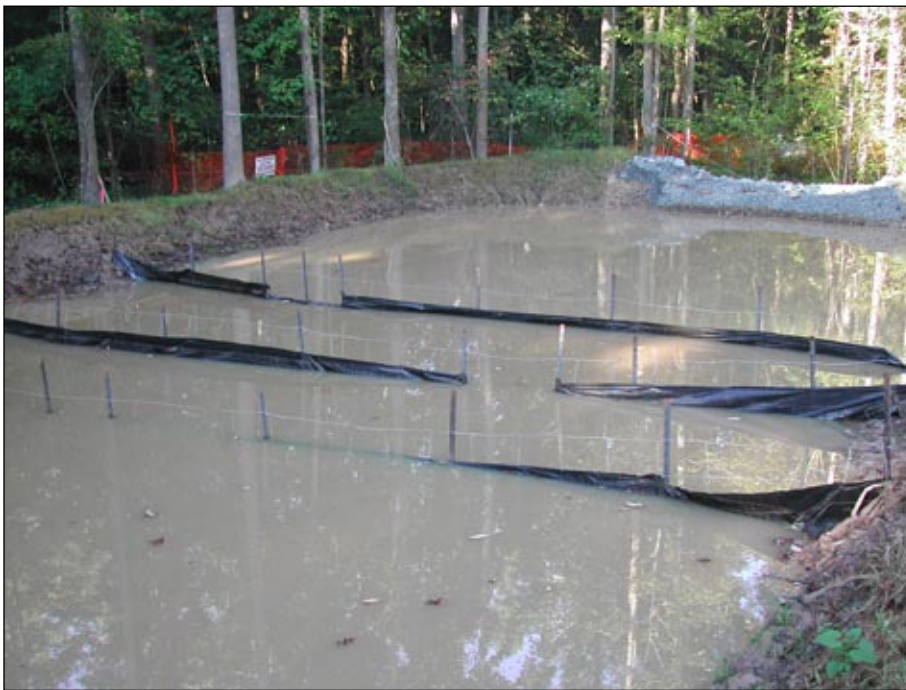
Figure 3. Example of silt fence with weirs cut at opposite sides to increase the flow path as the runoff moves toward the outlet.
