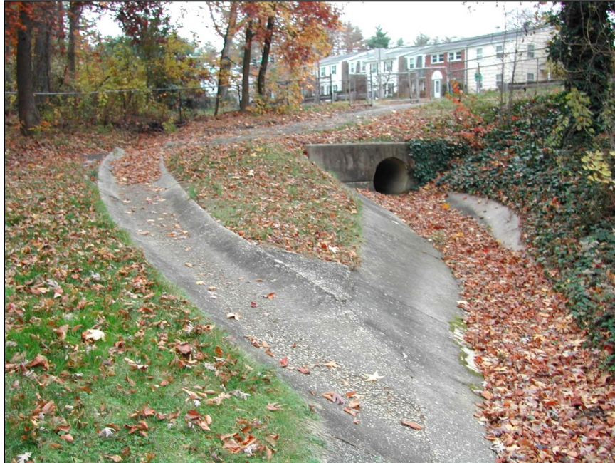
A stormwater outfall at Race Track Road in Bowie
